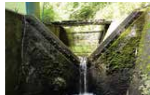
V-notch weir for observation of river flow discharge
